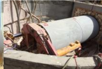
RC Jacking Pipes
